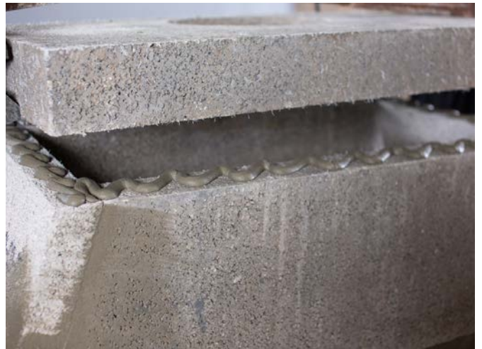
Apply lip glue to the top of the gather unit and then press the top plate into position with the hole offset closer to the rear section of the gather. Ensure the top section is level. Clean off any excess glue
