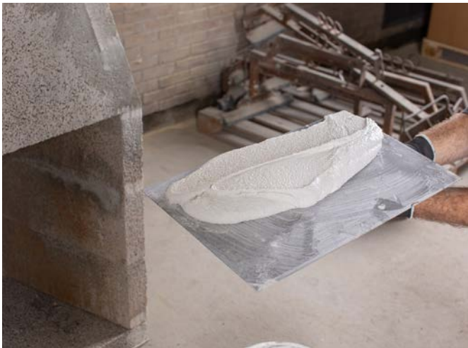
Mix the render as per the instructions on the bag.
