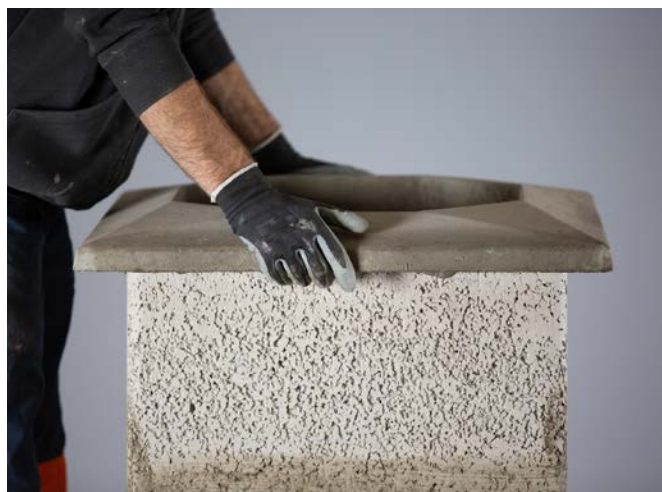
Glue on the capping.
