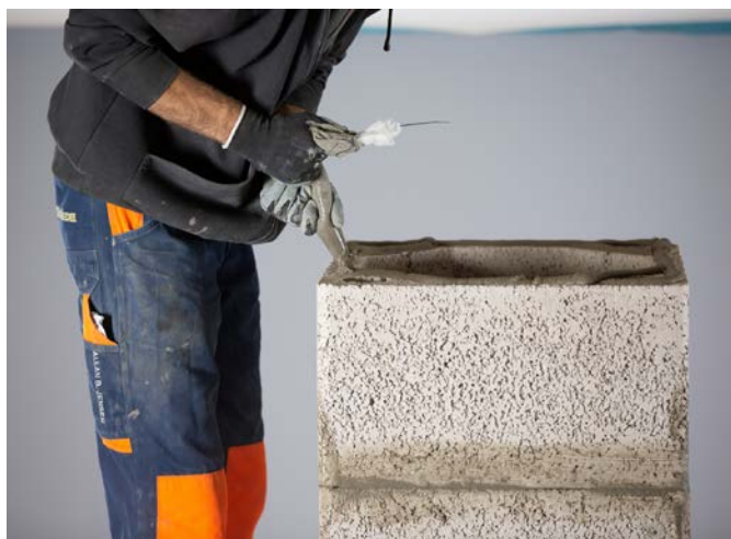
Glue on the next two chimney blocks.
